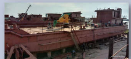
Fig 2 – Self propelled pipe carrying barge in Karnafuly Dockyard, Chittagong
